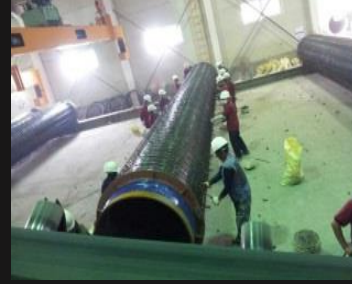
⑥ Spacer installation
