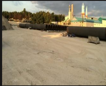
⑩ Final inspection (repair, ovality)
