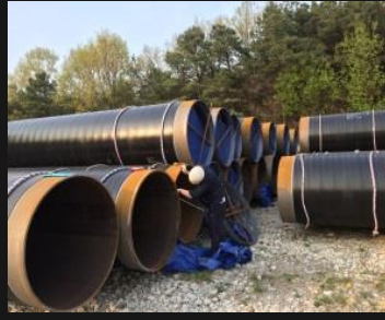
② Visual inspection (Ovality, PE coating)
