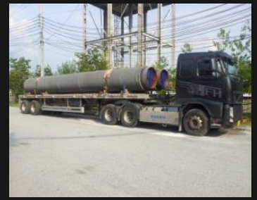
⑫ Pipe release
